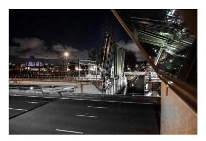
The Schinkelbrug is not operated from the towers anymore, but from the temporary site hut, where the operators to open the bridges remotely, using cameras. We call this 'remote operation'.
