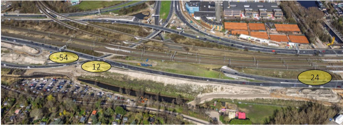
Work site for the installation of 66 piles and 24 dam walls
