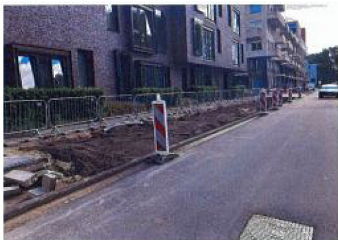
Part of the street that still needs to be paved.
